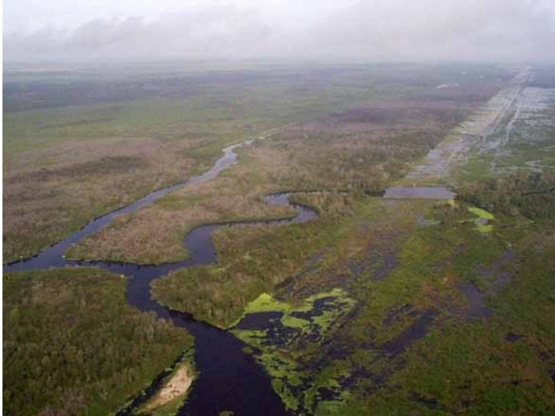
Figure 4-3. Restored portion of the Kissimmee River, Pool B/C. Remnants were left as is, recarved portions were dredged through former spoil deposits, and connectors go across backfilled C-38. Backfilled areas appear to have more ponding than the adjacent floodplain (Source: http://www.saj.usace.army.mil/dp/Kissimmee/Aerial_1.jpg ), although in time the difference may be reduced.
