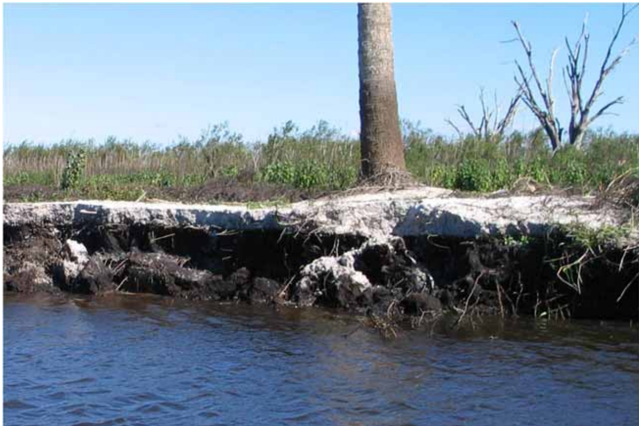
Figure 3-12. A sand splay 26 cm deep (levee building event), measured in December, 2008 between transect 3 and transects 4, 5, and 6. Photo credit: Edward Schenk, USGS.
