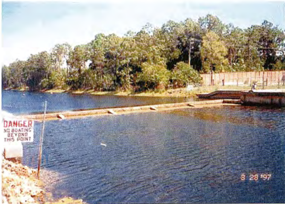
Figure 1-1: Existing Golden Gate Canal Weir No. 2
