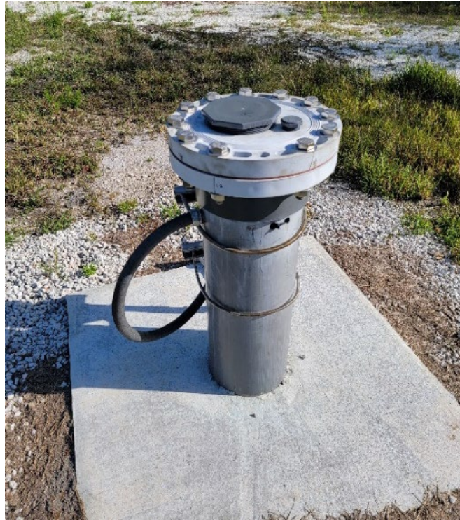
Figure 2. Wellhead configuration of OSF-99R.
