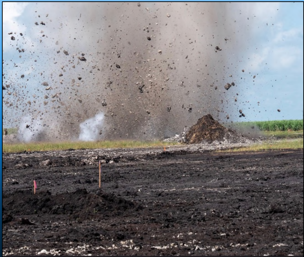
Recent Blasting at the EAA Reservoir Project Site
