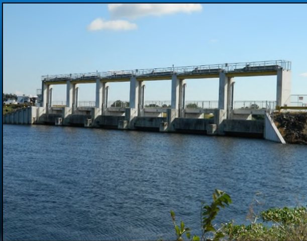
Water Control Structure
