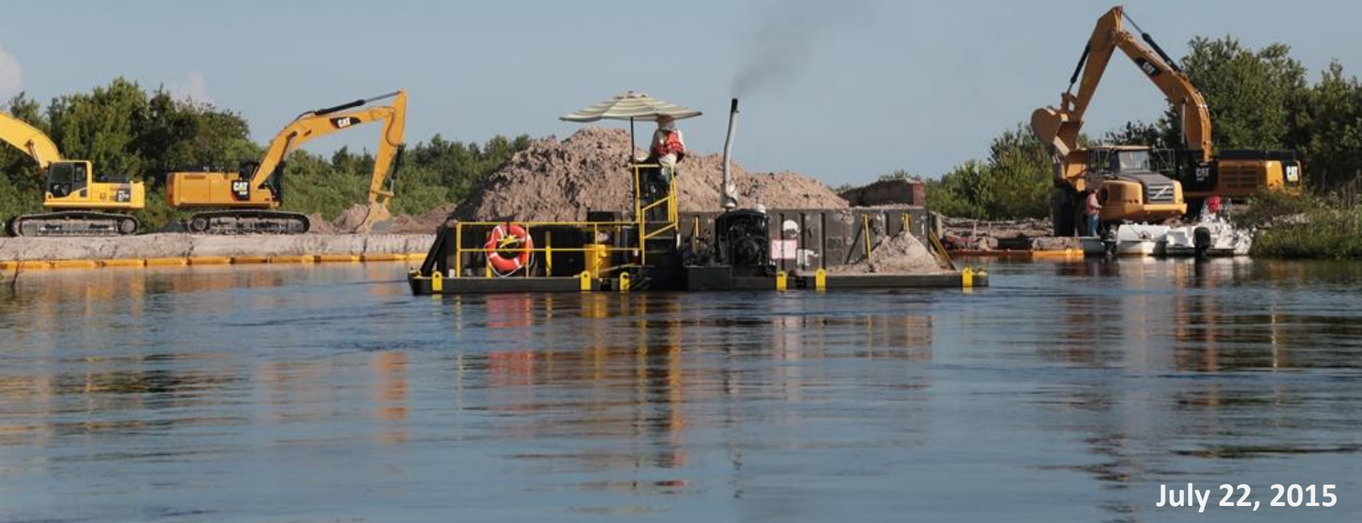
Construction of the Kissimmee River Restoration Project MacArthur Ditch contract continued through July as barges loaded down with fill made their way to the backfill area.
