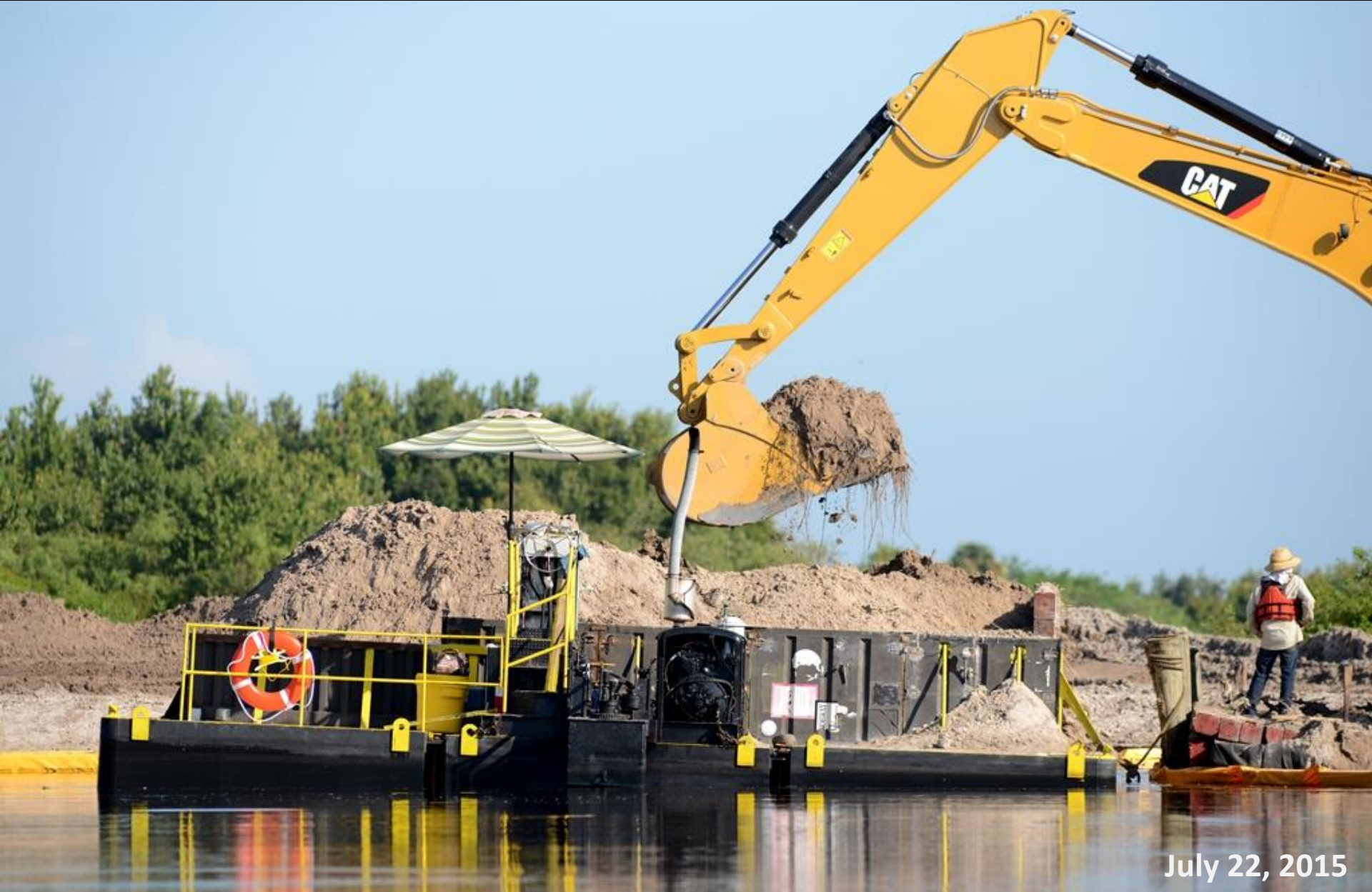
Excavators on the Kissimmee River Restoration Project MacArthur Ditch backfill project unload fill from a barge. Spoil is brought to the backfill site from spoil piles roughly 0.5 miles downstream long the C-38 canal.
