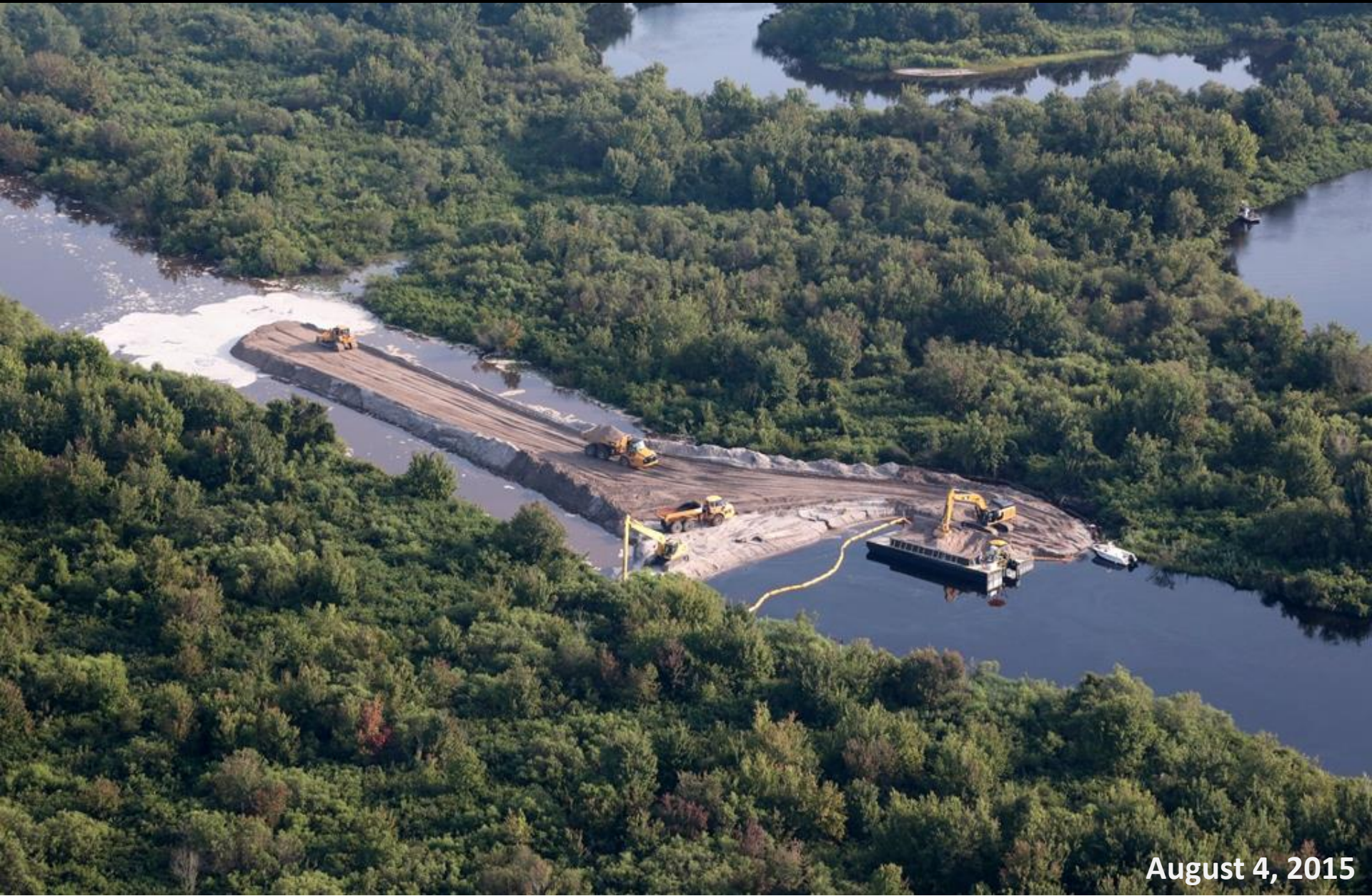
Looking at the construction of the MacArthur Ditch backfill project: A spoil plug has been placed across the south end of the ditch and the backfill continues northward into the Kissimmee River Restoration Project Phase I restoration area floodplain.
