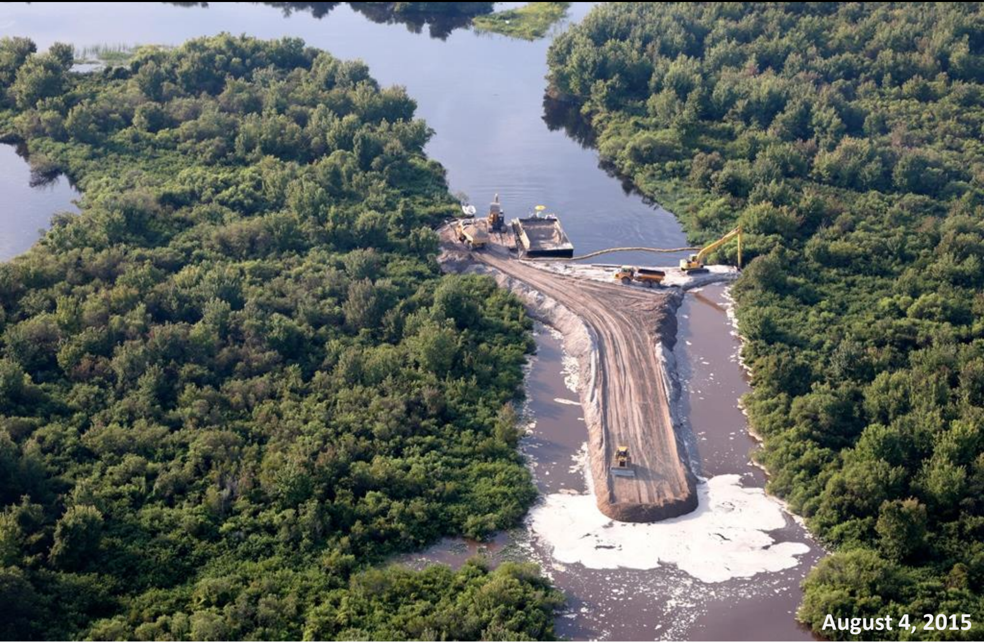
Looking south at construction of the MacArthur Ditch backfill project: The initial work of a spoil plug has been placed on the south end of the ditch and the backfill continues northward.
