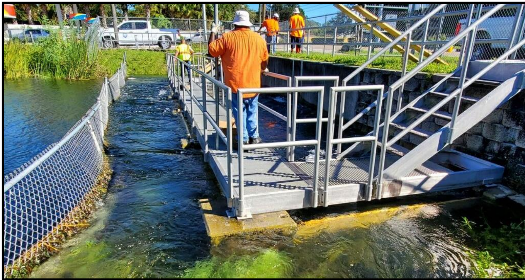
Chain-link Fence used as a Barriers
