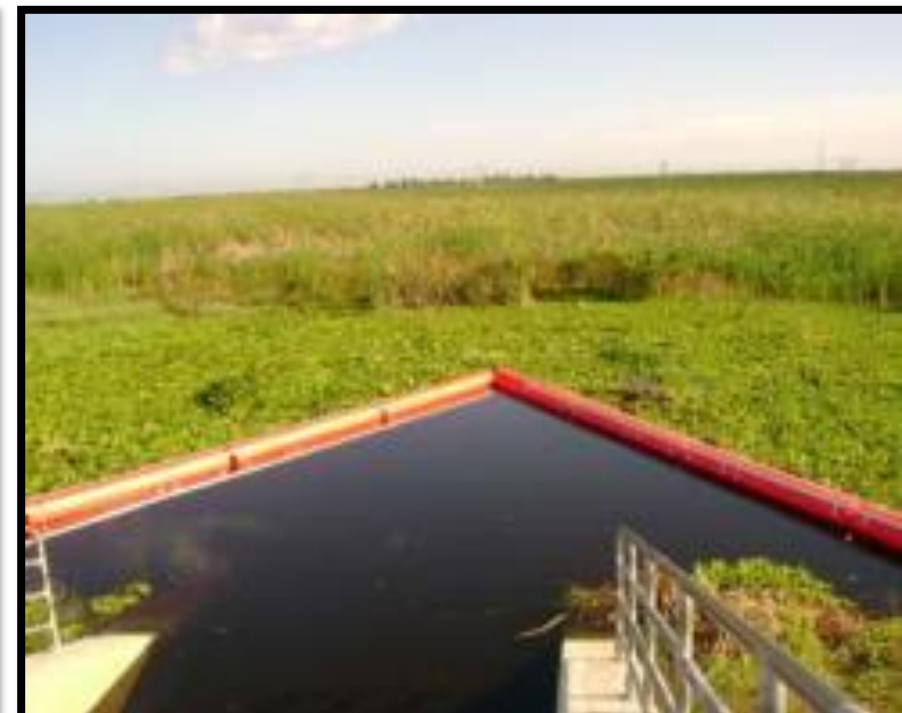
Water Control Structure
